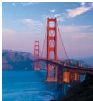
Golden Gate bridge
